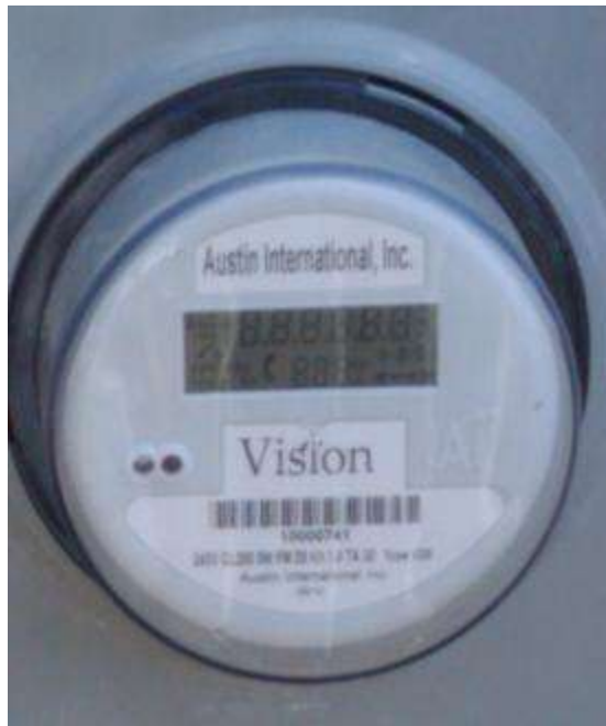
6. Closeup – Solar (REC) meter (meter make, model, kWh readout, and meter # visible)
